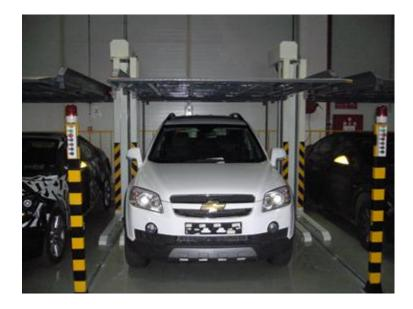
LARSSON also provided a PPY parking system for this project, PJS parking equipment is used on ground parking, which provided twice as many as ground car parking places.
