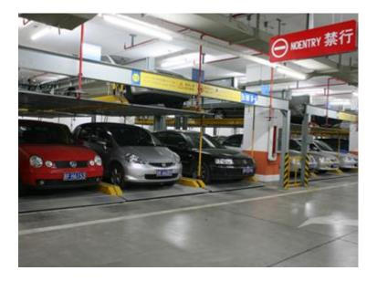
This Project is located in headquarters of CNC, 2 layers ad 3 layers of PSH parking equipments, total 472 car parking places, which is twice as many as initial designed ground parking places.
