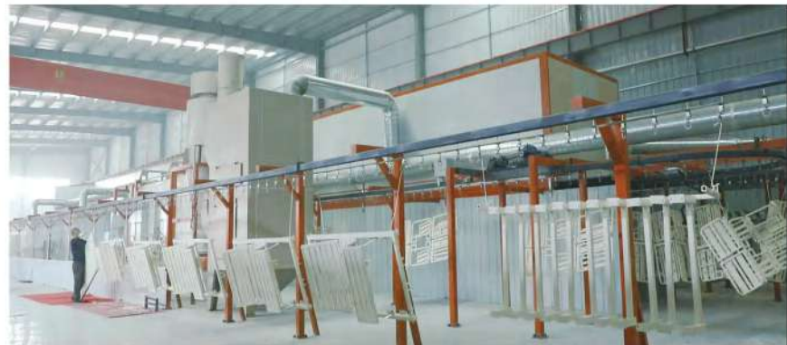
喷涂车间 Painting workshop
